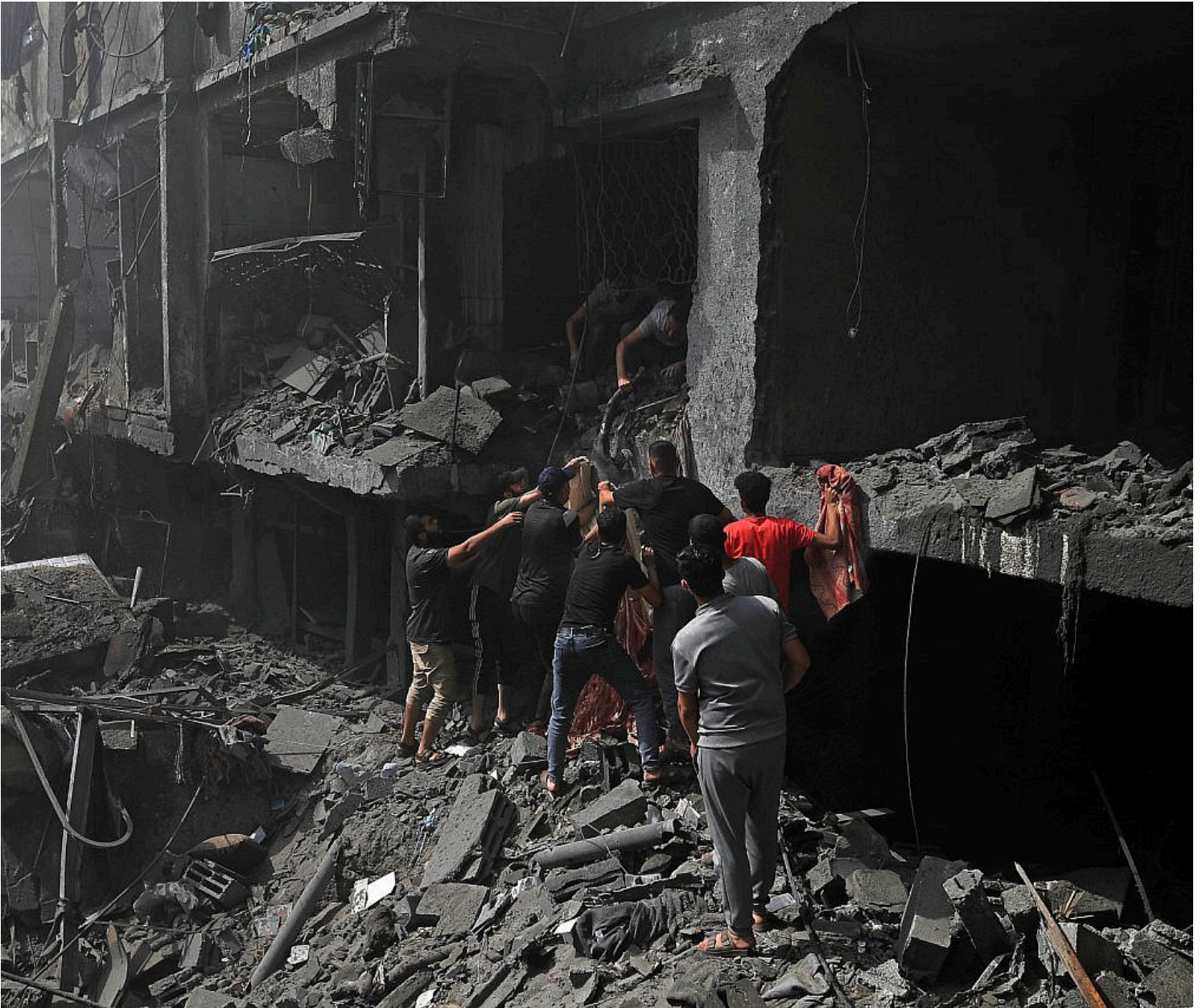
Survivors and bodies are pulled from the rubble after Israeli airstrikes hit buildings near Al-Aqsa Martyrs Hospital in Deir al-Balah, central Gaza, October 22, 2023. (Mohammed Zaanoun/Activestills)
